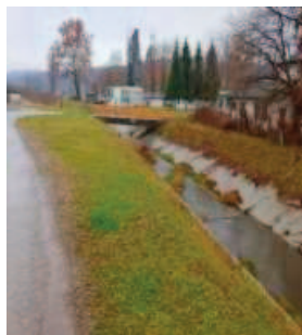
Figure 4. River Joševica, flows through compound PC RBC TUZLA INCUBATOR „LIPNICA“ D.O.O, the trough has been completely renovated - concreted along its entire length
