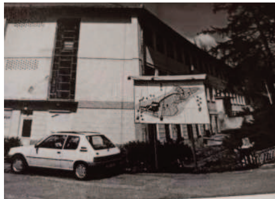
Figure 1. Administration building of the Lipnica mine - today the administration of the incubation centre
